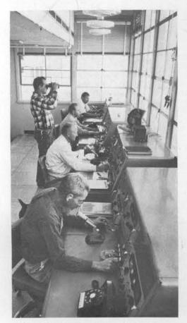
CONTROL POINT at Tonopah Test Range coordinates optical, electronic and telemetry systems to ensure that all are functioning properly as countdown progresses. Contact is also maintained with test aircraft. From top to bottom are: John Lindman, Ken Nielsen, R. R. Petrini (standing), Rush Robinett, and Fred Steele.
